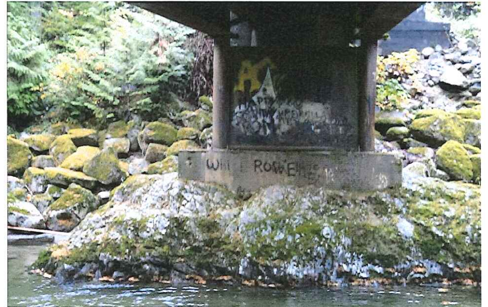
CK2107 Pier from Left
