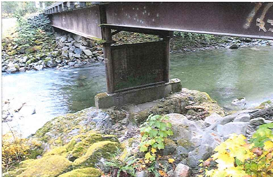
CK2107 Pier from Right
