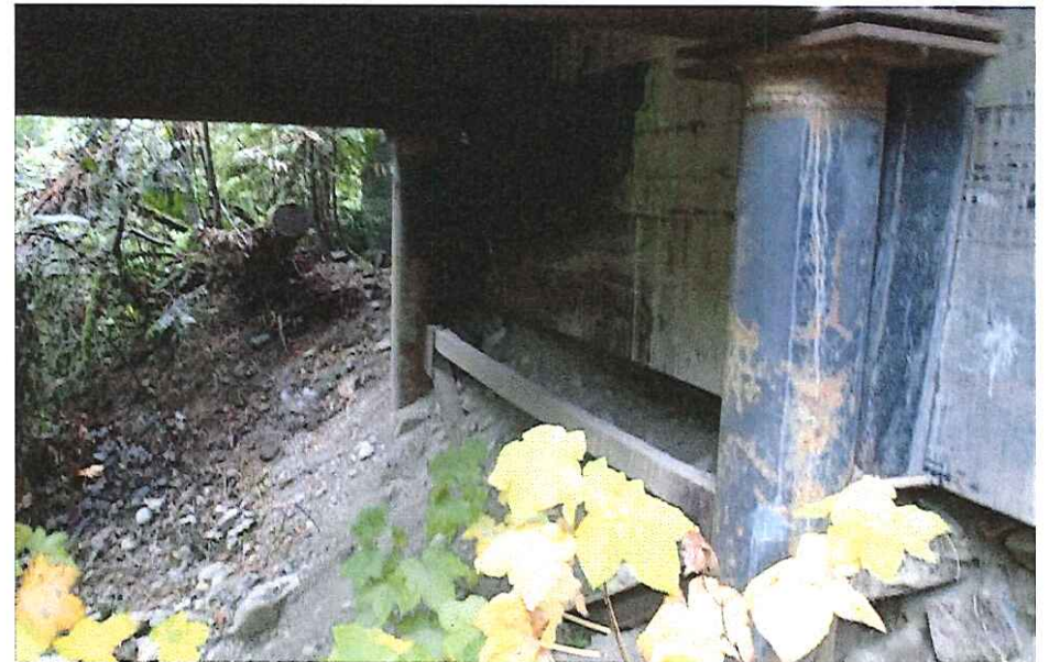
CK2107 Right Abutment
