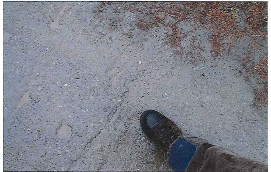
CK2107 Deck Joint
