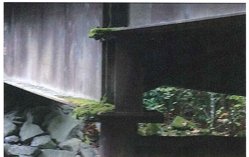
CK2107 Pier Bearing
