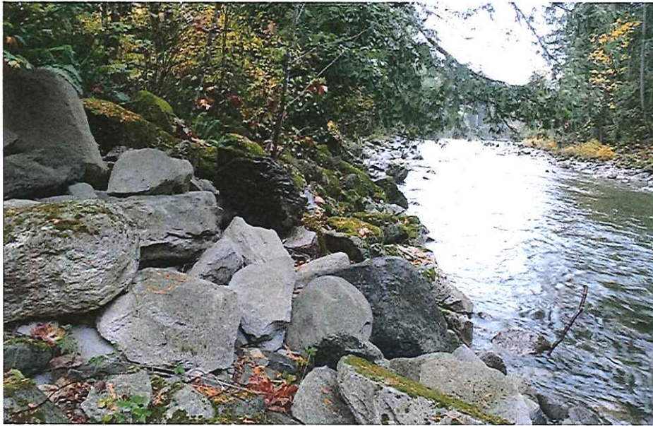
CK2107 Left Abutment Riprap
